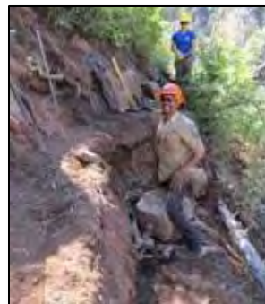
Heavy reconstruction on the Wilson Mountain National Recreation Trail.
