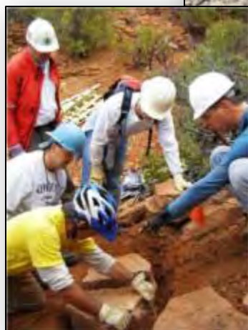
Verde Valley Cycling Coalition members armor the surface of a local trail.
