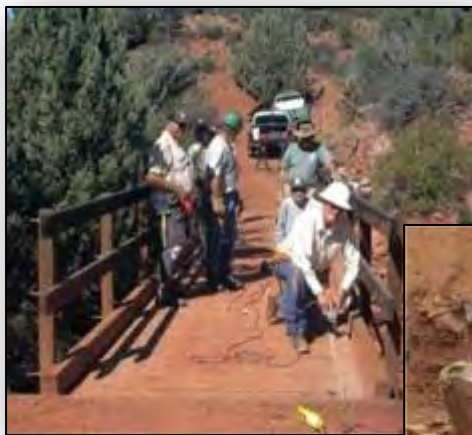
New decking on Bell Rock Pathway Bridge.
