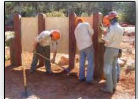
Rural Environmental Corp members finish installing a trailhead kiosk.
