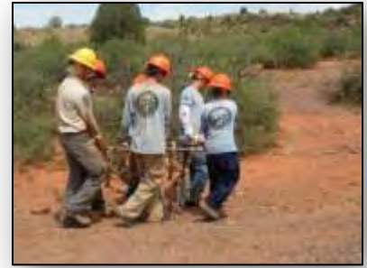
YCC youth move heavy rocks for the Walker Restoration Project.
